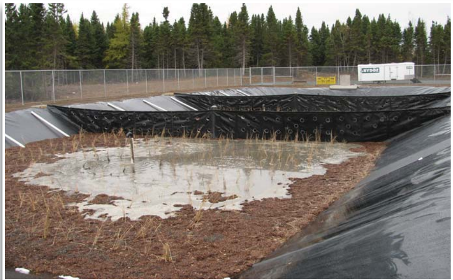
Figure 3. Sludge cells being filled at Appleton-Glenwood.
