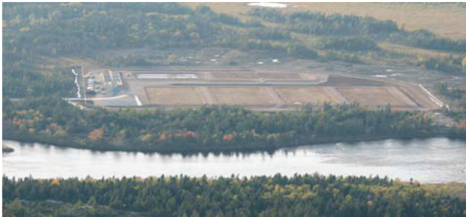
FIGURE 3. Aerial View of Appleton/Glenwood System—Spring 2007.
